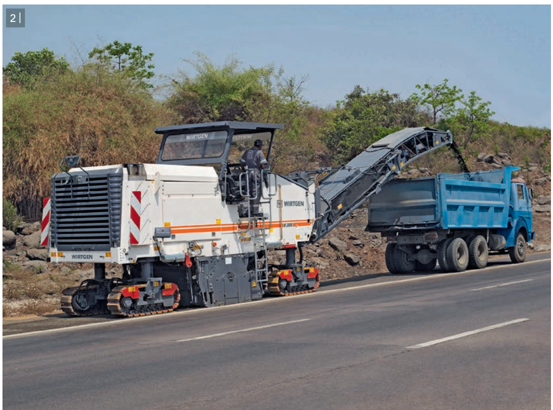
1-2 | The W 2000 large milling machine efficiently removes complete road pavements as well as individual pavement layers.
